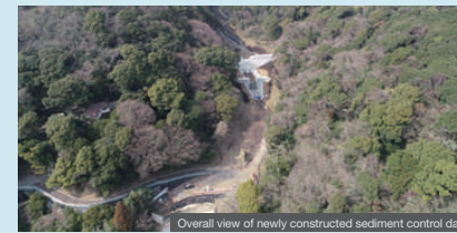
Overall view of newly constructed sediment control dam
