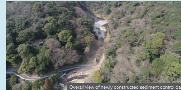
Overall view of newly constructed sediment control dam
