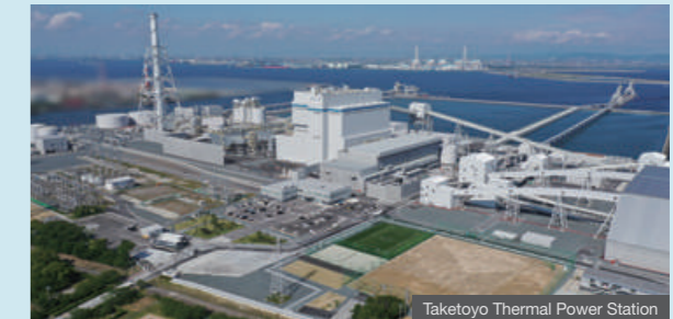
Taketoyo Thermal Power Station
