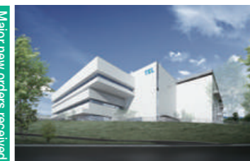
Tokyo Electron Miyagi Ltd. 3rd Development Building (Taiwa-Town, Kurokawa-gun, Miyagi Prefecture) Owner: Tokyo Electron Miyagi Ltd.
