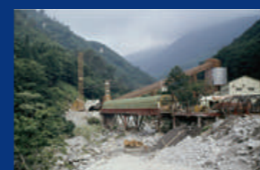
Joetsu Sinkansen Line Daishimizu Tunnel
