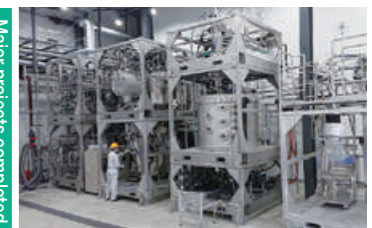
Construction of Takasago Chemical iFactory (Kakegawa-shi, Shizuoka) Owner: Takasago Chemical Corporation
