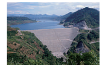
Cirata Hydroelectric Power Plant, Indonesia
