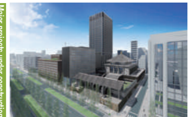
(Tentative name) Honmachi 4-Chome Project (Osaka-shi, Osaka) Owner: Taisei Corporation and Soai Gakuen * Joint development project
