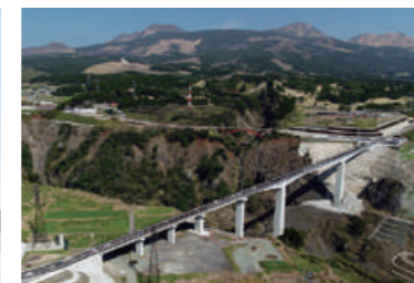
National Highway 325, Shin-Aso Ohashi Bridge
