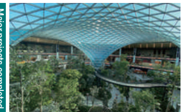
Hamad International Airport Expansion Project: Passenger Terminal Expansion Works—Central Concourse Building and Early Works (State of Qatar) Owner: Qatar Company for Airports Operation and Management (MATAR)
