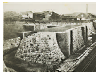
Lake Biwa Canal Sluice Gate
