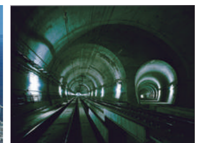
Seikan Tunnel [Yoshioka section]
