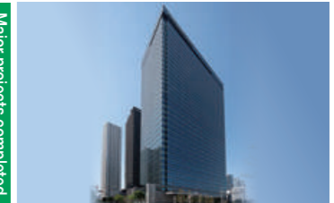
New Building Construction Work for Nishi-Shinjuku 5-chome Kita Project (Shinjuku-ku, Tokyo) Owner: Business Association of Nishi-Shinjuku 5-chome North Block Disaster Prevention Improvement Project
