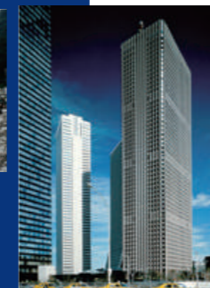
Shinjuku Center Building
