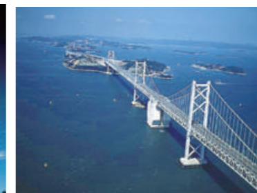
Minami & Kita Bisan-Seto Bridges [substructure, North segment]
