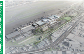
Fukuoka Airport International Terminal Buildings, Extension and Renovation Work (Fukuoka-shi, Fukuoka) Owner: Fukuoka International Airport Co., Ltd.
