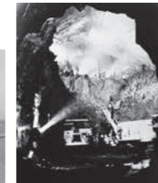
Kansai Electric Power Co., Inc., Kurobegawa No.4 Hydropower Plant [5th segment]
