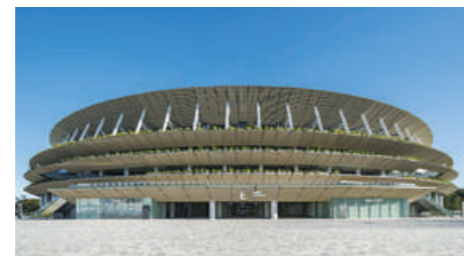
Japan National Stadium
